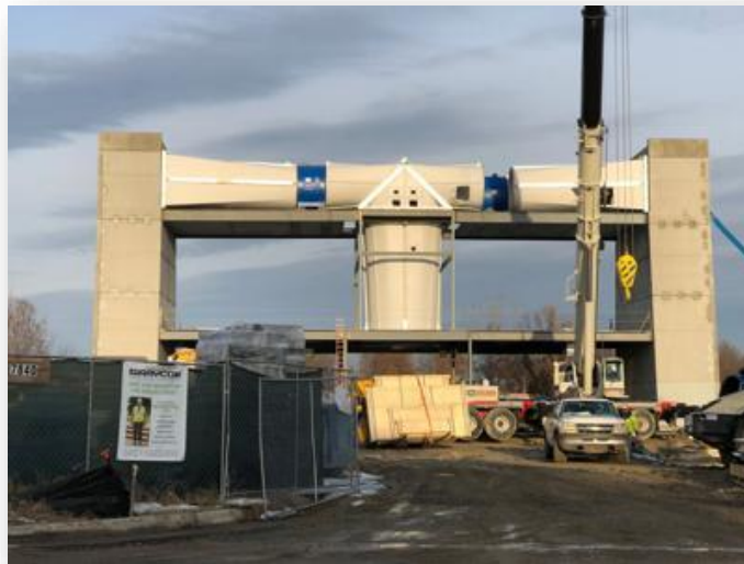
Model Gen 8 - 12R4 Under Construction
